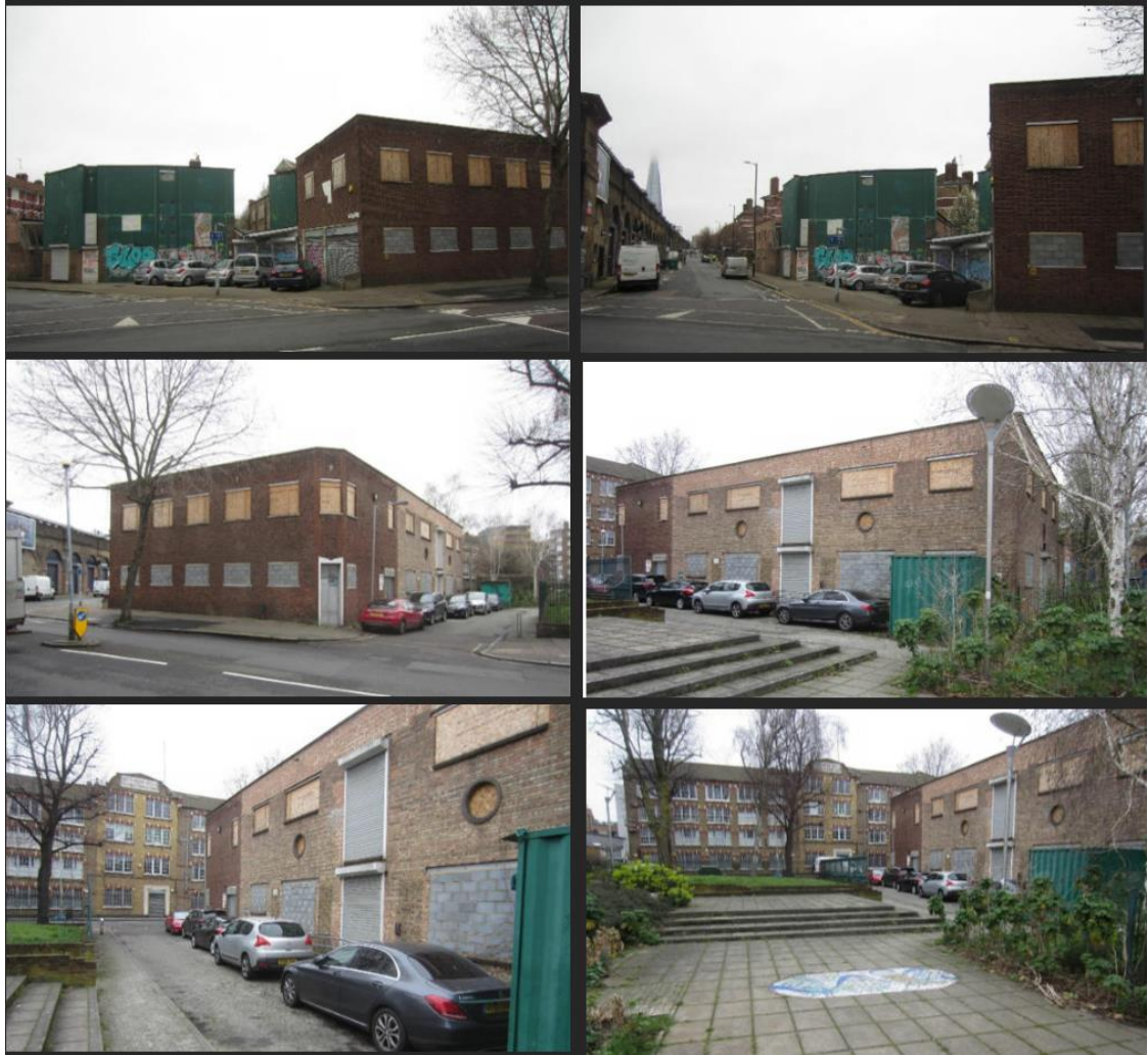
Image 08 (above): Images of the existing site prior to demolition, (clockwise from top left), view of site from corner of Druid Street and Abbey Street (top row), from Abbey Street (middle left), view of the existing site from Neckinger Street/open space (middle right, and bottom row).
